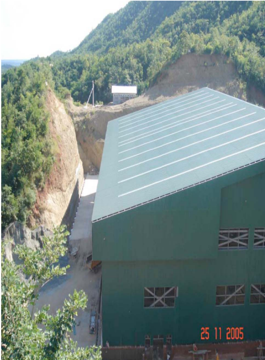
Figure 5. Factory 2 under construction in a photo provided by STW
